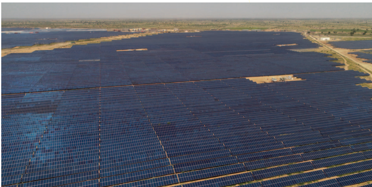
200 MW, Bhadla, Rajasthan.
