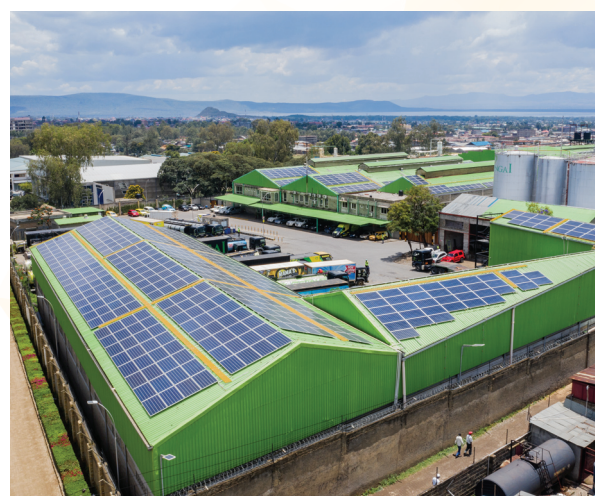
Aerial view of the 850 kW rooftop system.
