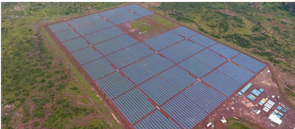
Kita, with a capacity of 50 MW the largest solar power plant in West Africa.
