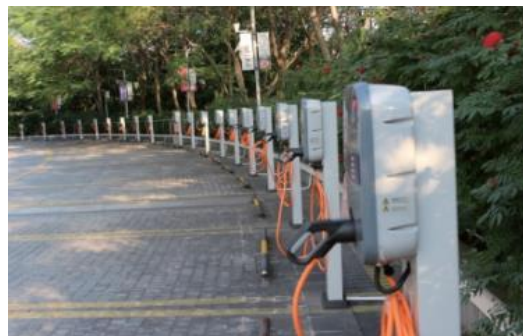
YOHO Bay Project
