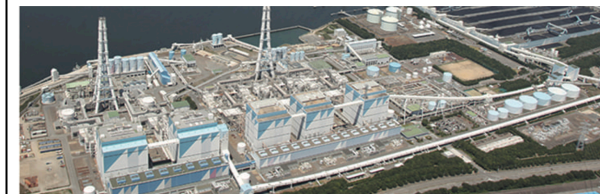
1. JERA's 4.1-GW Hekinan Thermal Power Station is one of the world's biggest coal plants. The plant houses five units. Units 1, 2, and 3 are 700-MW units that opened between 1991 and 1993, and Units 4 and 5, 1 GW each, opened in 2001 and 2002. Courtesy: JERA
